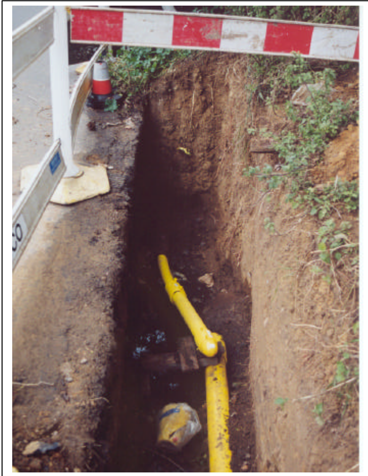
Photograph No 7 Lower trench from which soil and root samples were taken.
