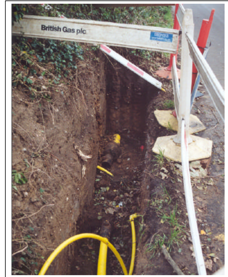
Photograph No 8 Upper trench from which soil and root samples were taken.
