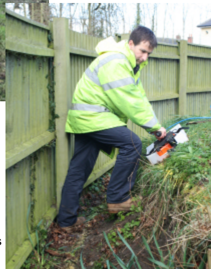
Hand use of GPR on banks
